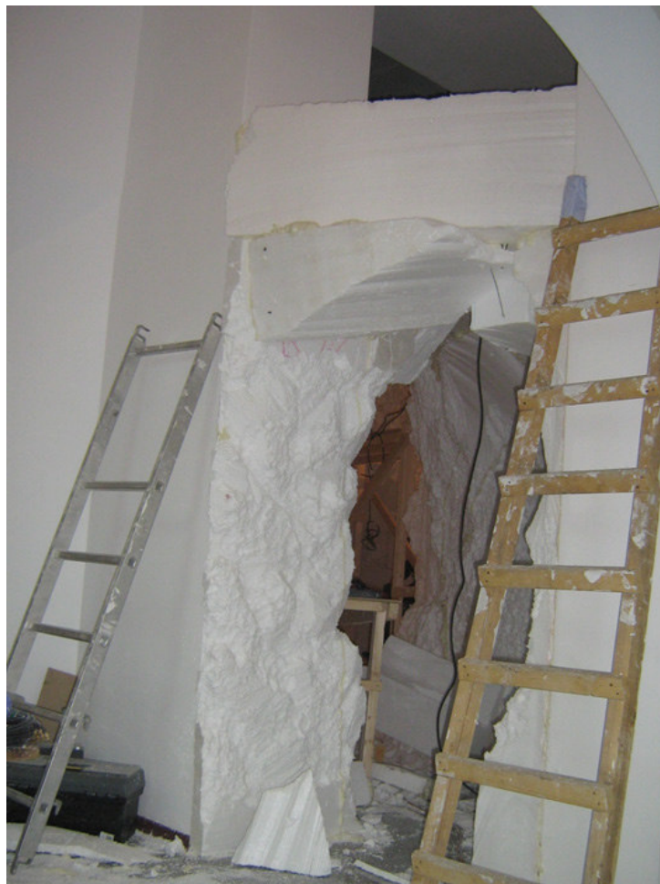
Fig. 1: The installation of the polystyrene blocks and their carving (original).
